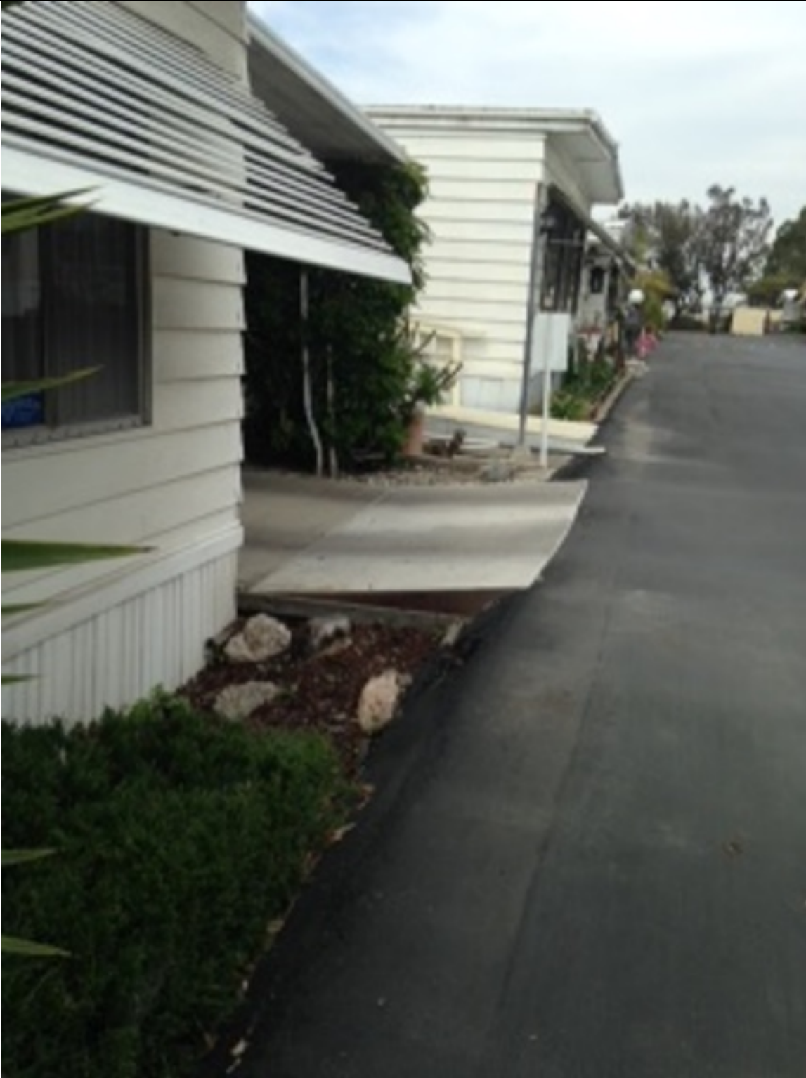
Picture of violation G/O-3
